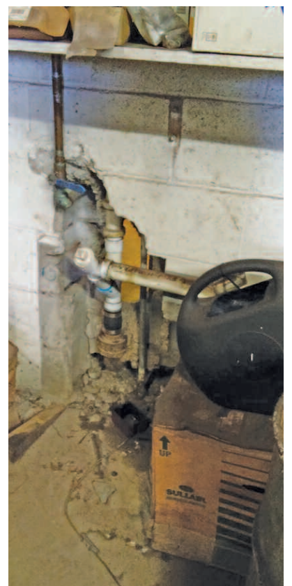
Broken pipes are a common sight through the DPW and Fire Garage where cracked cement and out of date equipment abound.
